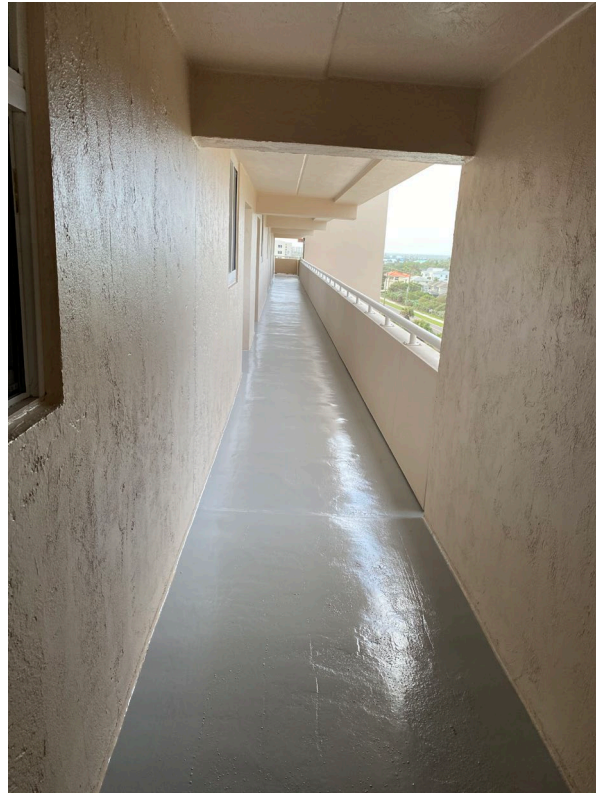
Picture 5: Base coat application on the 6 th floor walkway
