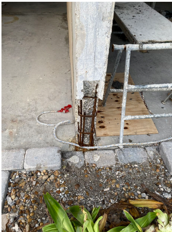
Picture 3: Typical wall repair
