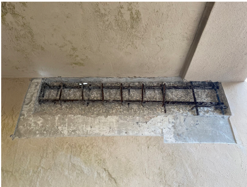
Picture 4: Typical wall repair
