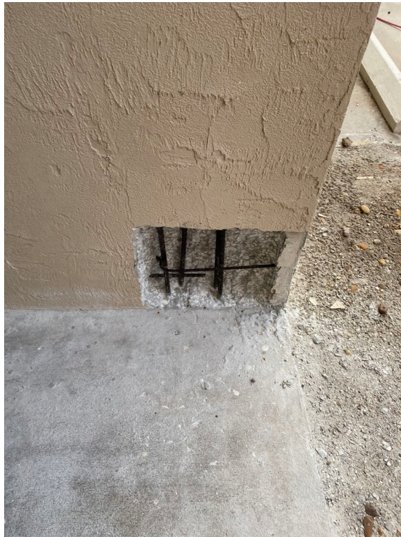
Picture 2: Typical wall repair
